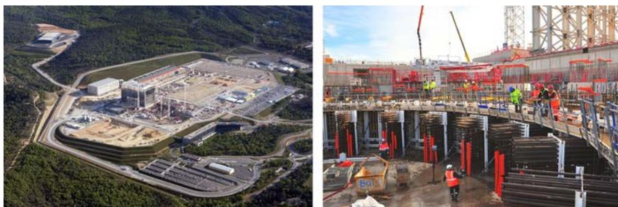
*FIG. B.6. Aerial view of the ITER construction site in August 2015 (left). As of 21 October 2015 (right), the 200° segment of the ITER bioshield, the 3.2 metre thick 'ring' that will surround the machine, was constructed. (Photographs courtesy of ITER.)*
