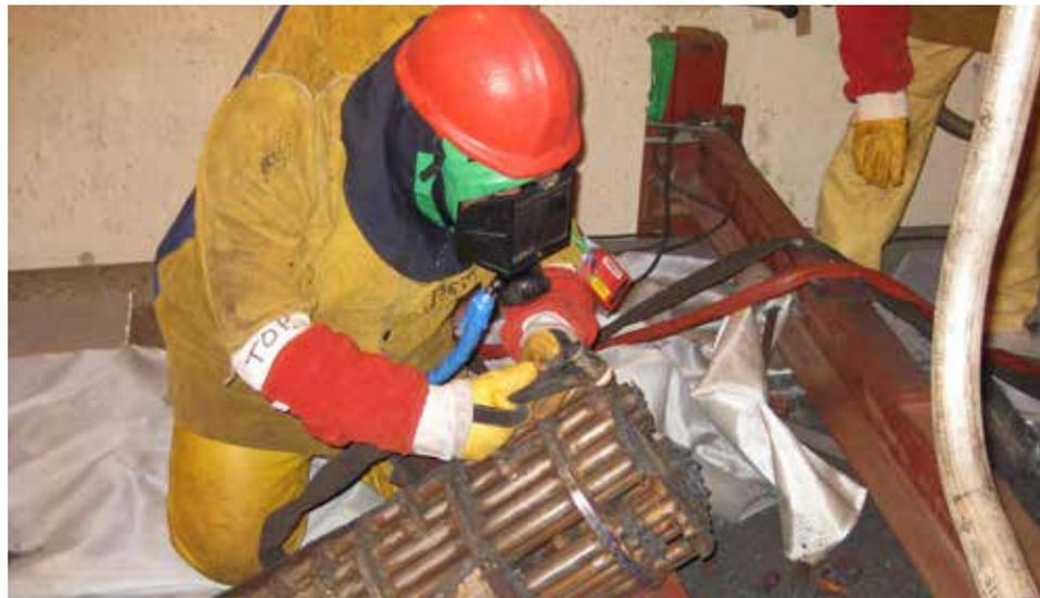
allows for easier breakdown of hard-to-reach and often radioactive parts. This prevents any direct contact by the operator, which in turn minimizes a person's exposure.
