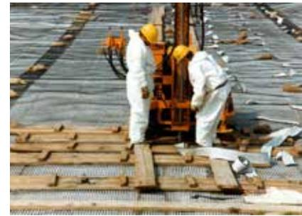
**Application of a combined scheme for covering and draining uranium mill tailings.**
