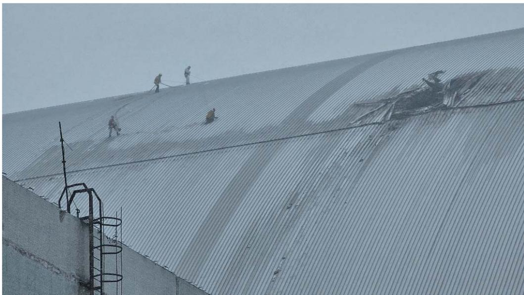
*Response personnel scale the NSC on 14 February 2025 as part of efforts to prevent fires spreading within the outer and inner cladding.*
