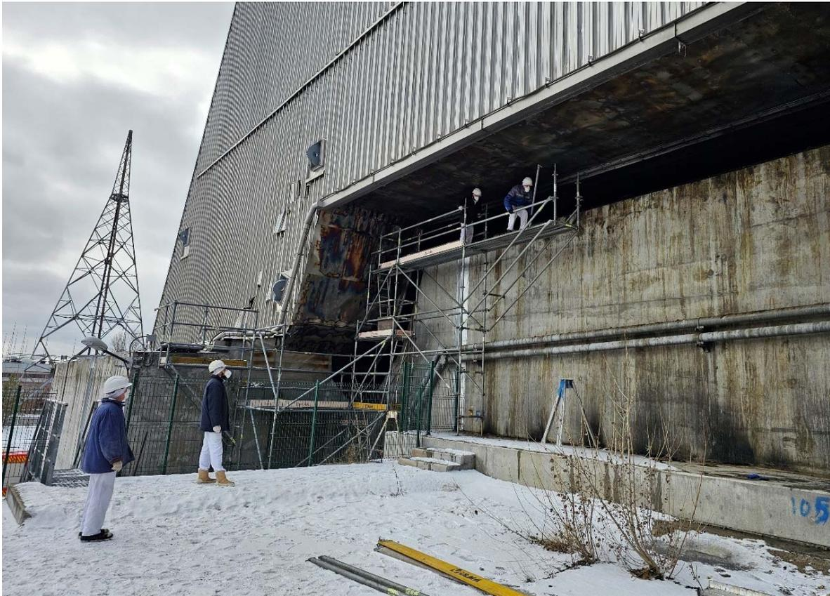
*Personnel inspecting damage to the membrane between the arch contour and the concrete support structure of the NSC on 20 February 2025.*
