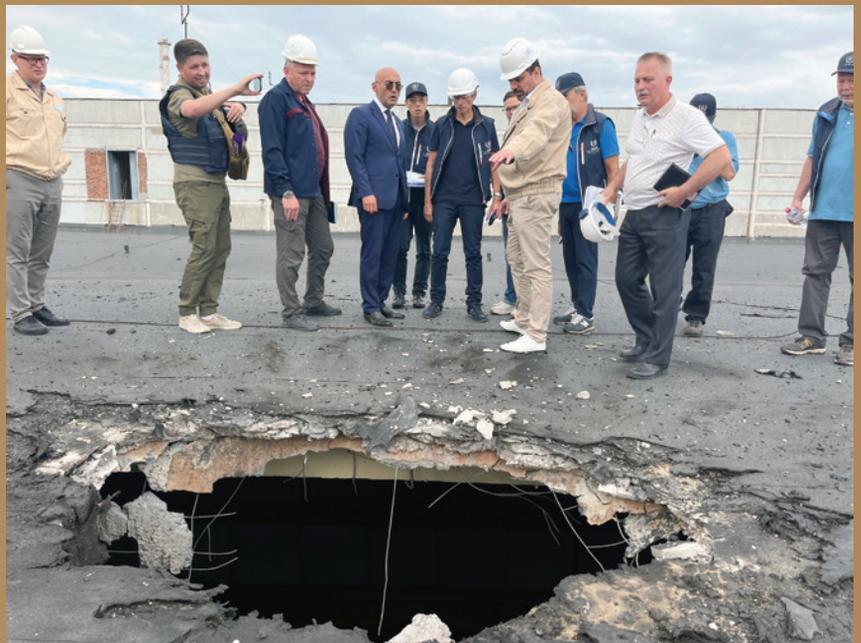
The IAEA team observes the damage caused by shelling on the roof of the special building at the ZNPP that houses, among other items, the fresh nuclear fuel and the solid radioactive waste storage facility. (Photo: IAEA)
