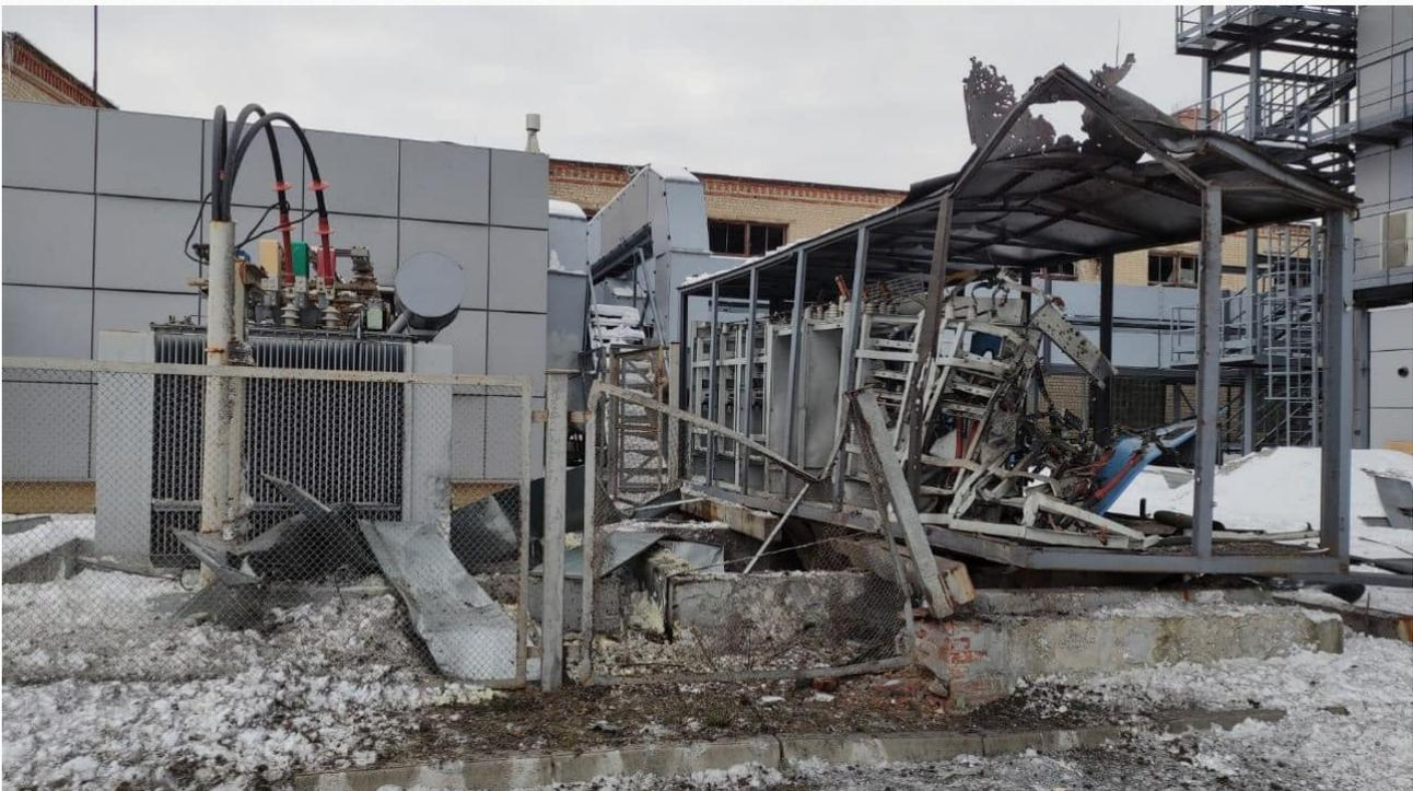
**Destroyed substation RU-0.4 kV.**
