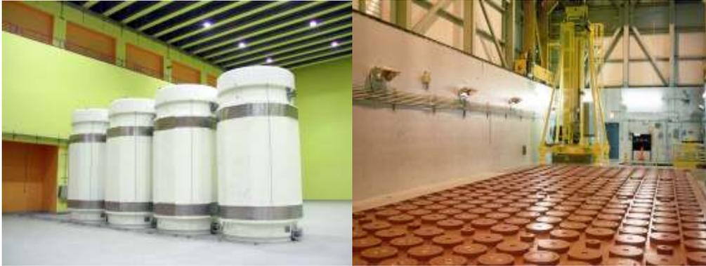
Figure 2. Dry fuel storage technologies: casks at the ZWILAG facility in Switzerland (left) and the Fort St. Vrain vault in the USA (right).
