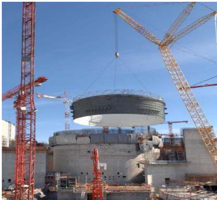
*FIG. IV-3. Lifting the containment liner double rings at Olkiluoto-3 in Finland.*
