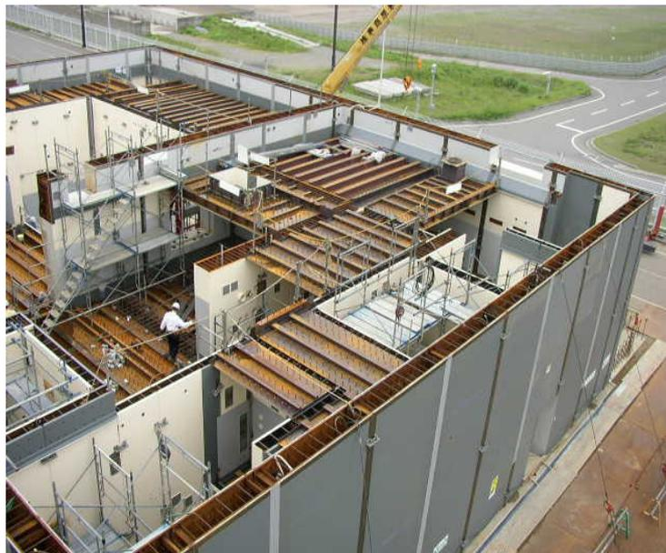
*FIG. IV-11(b). Steel Plate Reinforced Concrete*
