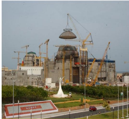
*FIG. IV-4. Lifting the WWER-1000 containment dome into position at Kudankulam, India (Photo credit: NPCIL).*
