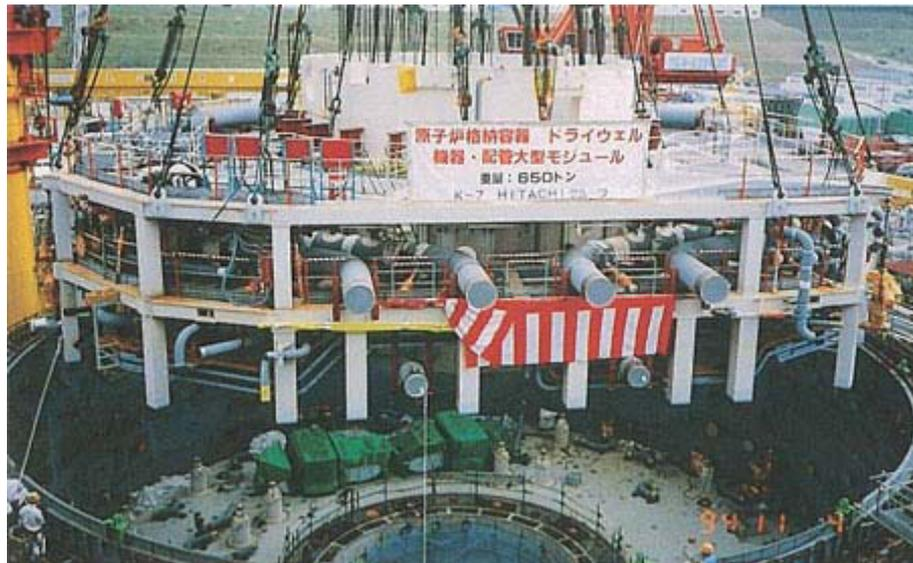
*FIG. IV-7. Installing the upper drywell super large scale module at Kashiwazaki Kariwa-7 in Japan.*
