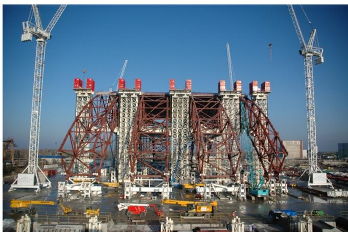
*FIG. A-18. The assembly of the new safe confinement for the fourth unit at the Chernobyl NPP (Photo: Chernobyl NPP).*
