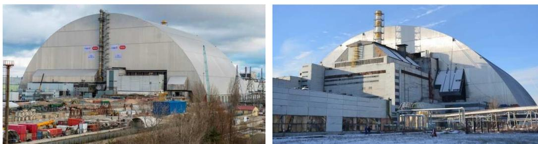
*FIG. A-6. The New Safe Confinement over Unit 4 of the Chernobyl NPP (left, view from the construction site; right, view from Unit 3). The structure is 108 metres high, 162 metres long and 257 metres wide, and weighs about 36 000 tonnes. (Photos: Chernobyl NPP)*
