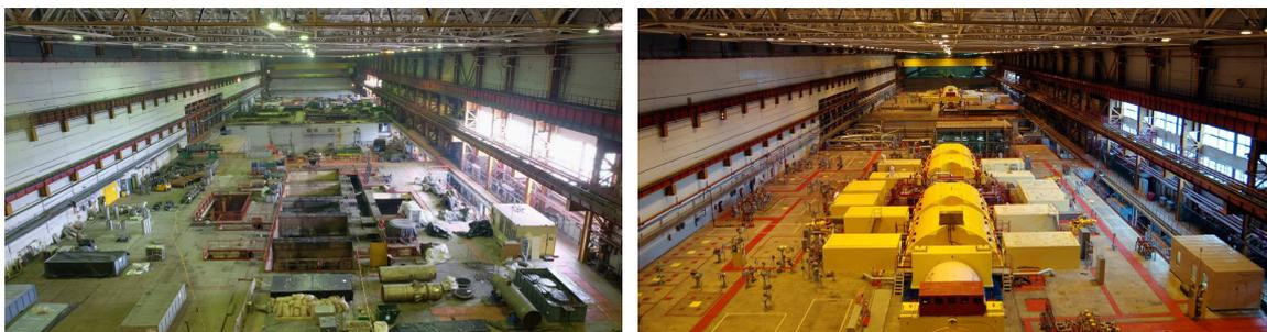
FIG. A-7. Dismantling activities at turbine halls of Units 1 (left) and 2 (right) of Lithuania's Ignalina NPP (Photos: Ignalina NPP).
