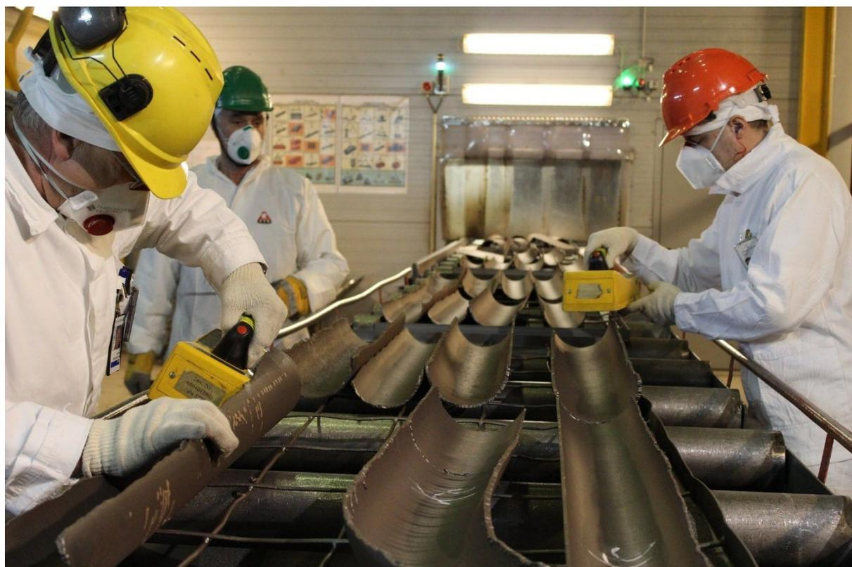
*Workers dismantling the Turbine Hall at Ignalina Nuclear Power Plant measure scrap metal for traces of radiation (Photo: J. Donovan/IAEA)*
