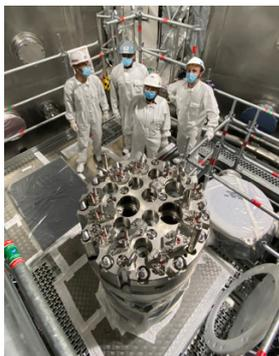
FIG. D-1 b. Installation of the closure head of the Jules Horowitz Reactor in Cadarache, France. (Photo: CEA).
