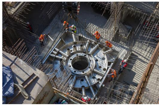
FIG. D-1 c. Installation of floor slab in the base of the MBIR reactor cavity, Research Institute of Atomic Reactors State Scientific Centre, Dimitrovgrad, Russian Federation. (Photo: Rosatom)
