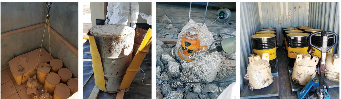
FIG. C-4. Retrieval and conditioning of radioactive sources in new waste packages at a legacy waste storage site in Jordan. (Photos: Jordan Atomic Energy Commission)
