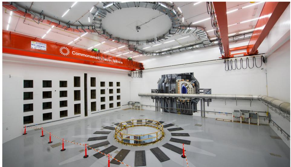
FIG. D.2. The SPARC tokamak hall ready for machine assembly. (Source: CFS)
