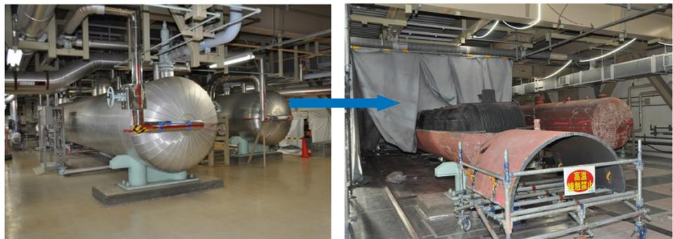
FIG. C.2. Dismantling a high-pressure feedwater heater as part of the decommissioning of the Monju reactor. (Source: JAEA)
