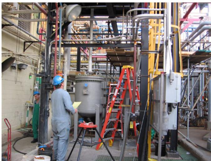
*FIG. A.10. New hydrogen fluoride vaporizer; Honeywell Metropolis Works facility, Illinois, United States of America (courtesy of Converdyn).*
