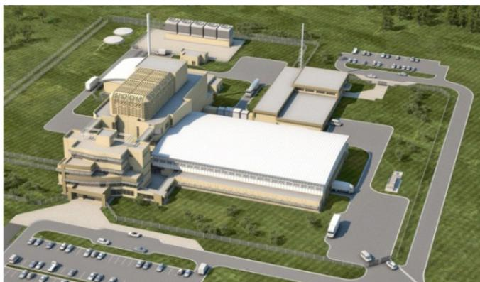
*FIG. C.3. Argentina's Nuclear Regulatory Authority has granted a construction licence for the RA-10 research reactor, which will be used to increase the country's production of radioisotopes for materials/fuels testing, doping of silicon, as well as R&D. (Image: National Atomic Energy Commission.)*
