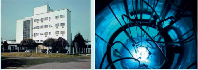
RA-3 reactor building (left) and reactor core during operation (right)
